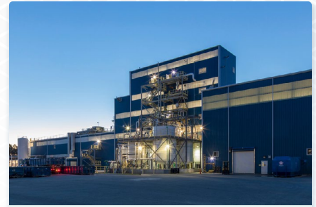
The Kings Mountain Lithium Conversion Facility: this facility transforms essential lithium resources into critical ingredients for mobility, energy, connectivity and health.
