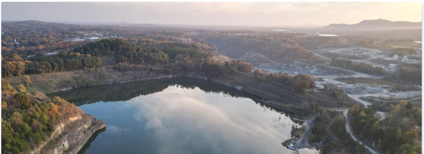
Kings Mountain Mine Site: The Kings Mountain Mine is expected to provide Martin Marietta's nearby quarry (shown here just beyond the existing mine pit) with non-ore-bearing material from the Kings Mountain Mine to process and sell as construction aggregate.
