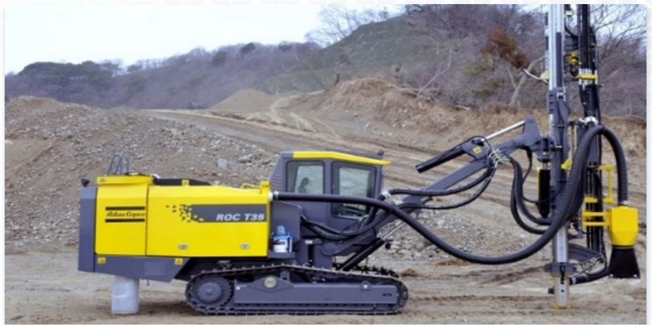
To prepare for blasting operations, a series of holes are drilled into the rock and then filled with an explosive.
