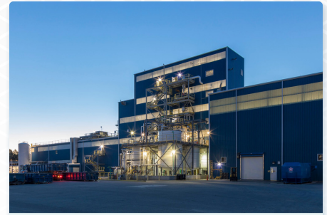
The Kings Mountain Lithium Conversion Facility: this facility transforms essential lithium resources into critical ingredients for mobility, energy, connectivity and health.
